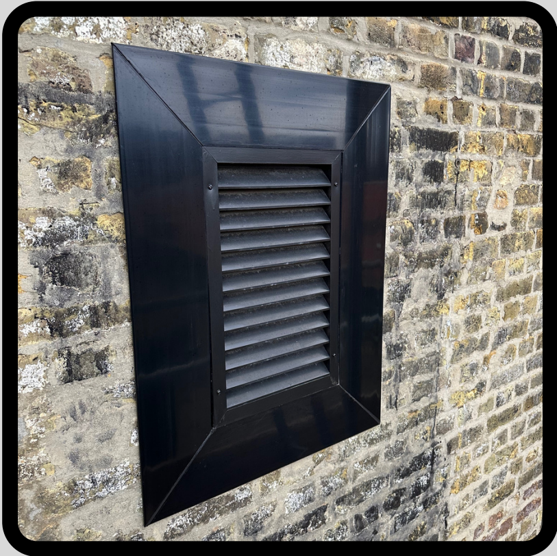
HVAC vents finished to prevent water ingress
