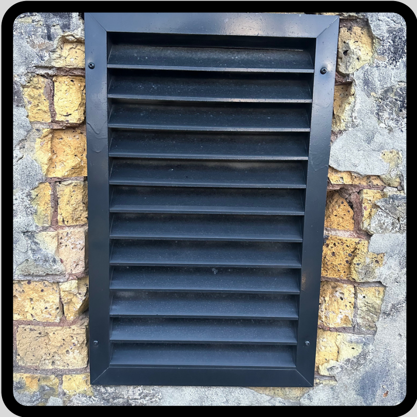
HVAC vents finished to prevent water ingress
